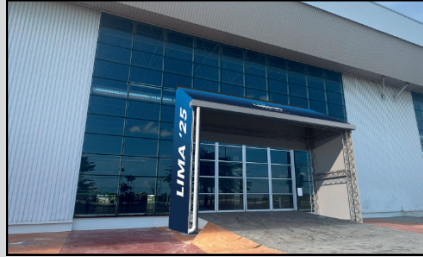
1 x Awning entrance at Hall A (View from Outside) Size: 9.5m (W) x 10.8, (Ht.)
